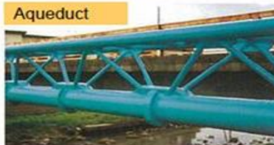
Additional pipes using bridge
